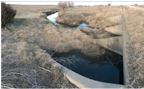
Figure 1.2 Example of silted culvert (structure code: 165881) in South-West Iowa
