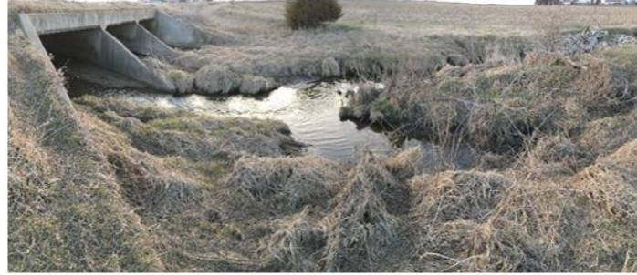
Figure 1.2 Example of silted culvert (structure code: 165881) in South-West Iowa
