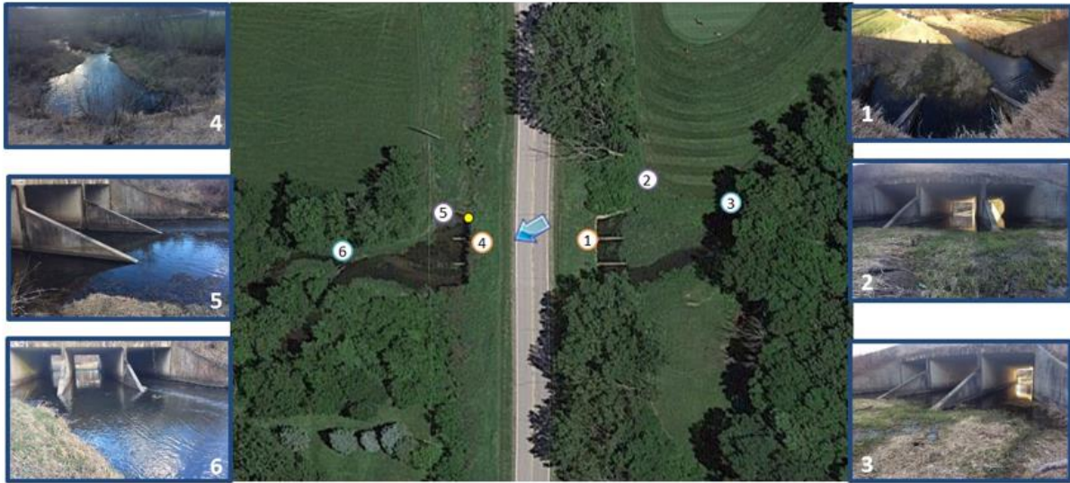
Figure 3.3 Field measurement protocols: a) positioning of the photo camera for the survey; b) illustration of the measurement acquired for the degree of sedimentation blockage; and c) illustration of the photo-documentation acquired at the culvert site
