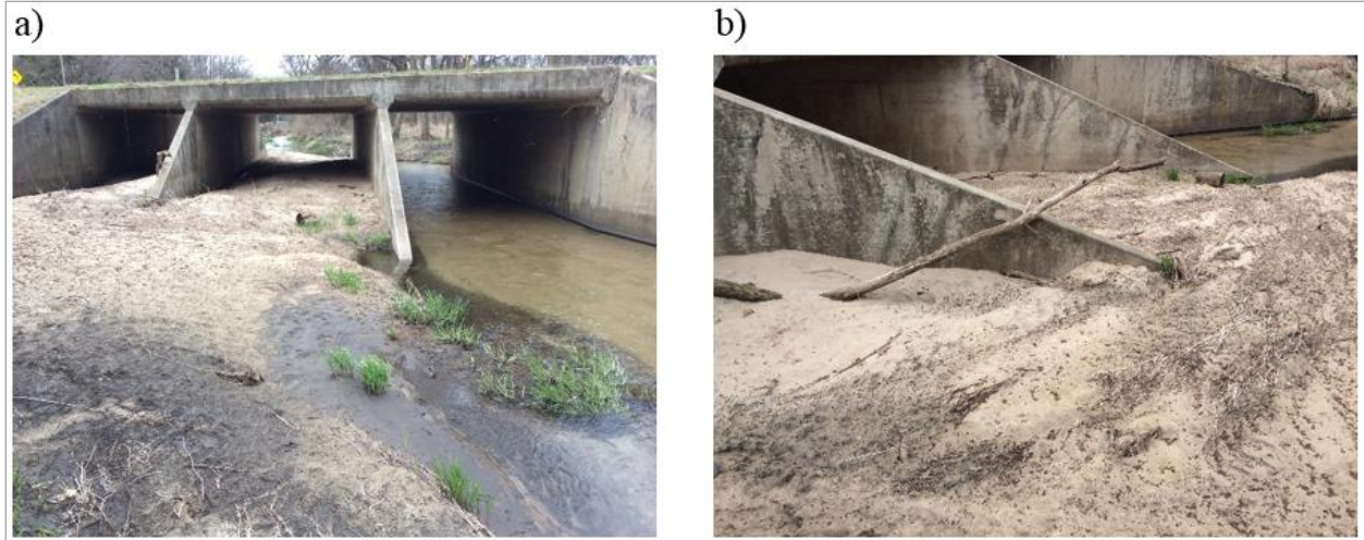
Figure 2.6 Fine-grained sediment deposits at culvert (structure code: 75050): a) the sediment deposited at the culvert was accumulated over 5 years; b) the absence of abundant vegetation development due to the nature of the substrate made of well-sorted quartz
