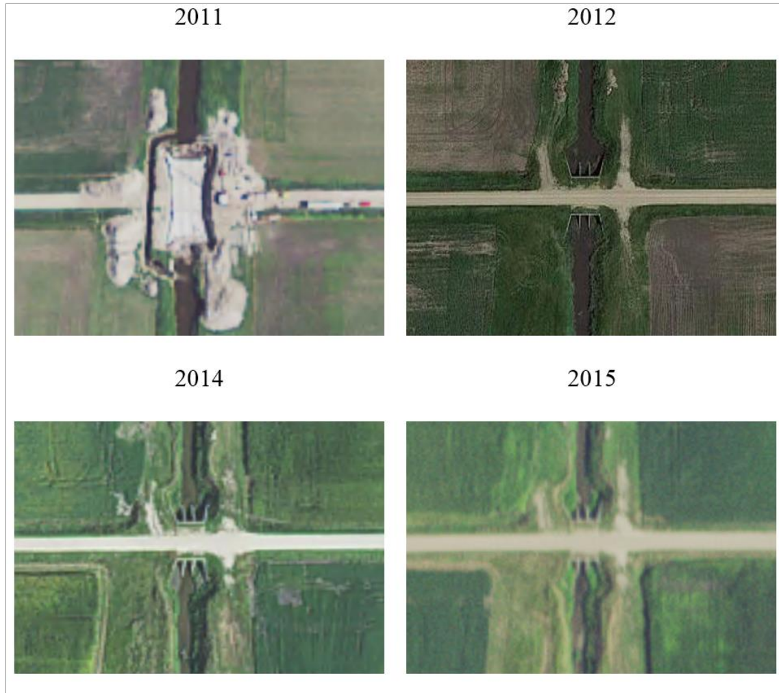
Figure 1.4 Sediment deposition at culverts is a fast process, impairing culvert's conveyance capacity in few years from construction completion (structure code: 344691)
